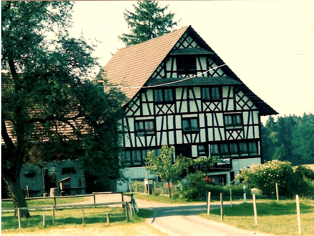
Untere Siten (front view)
