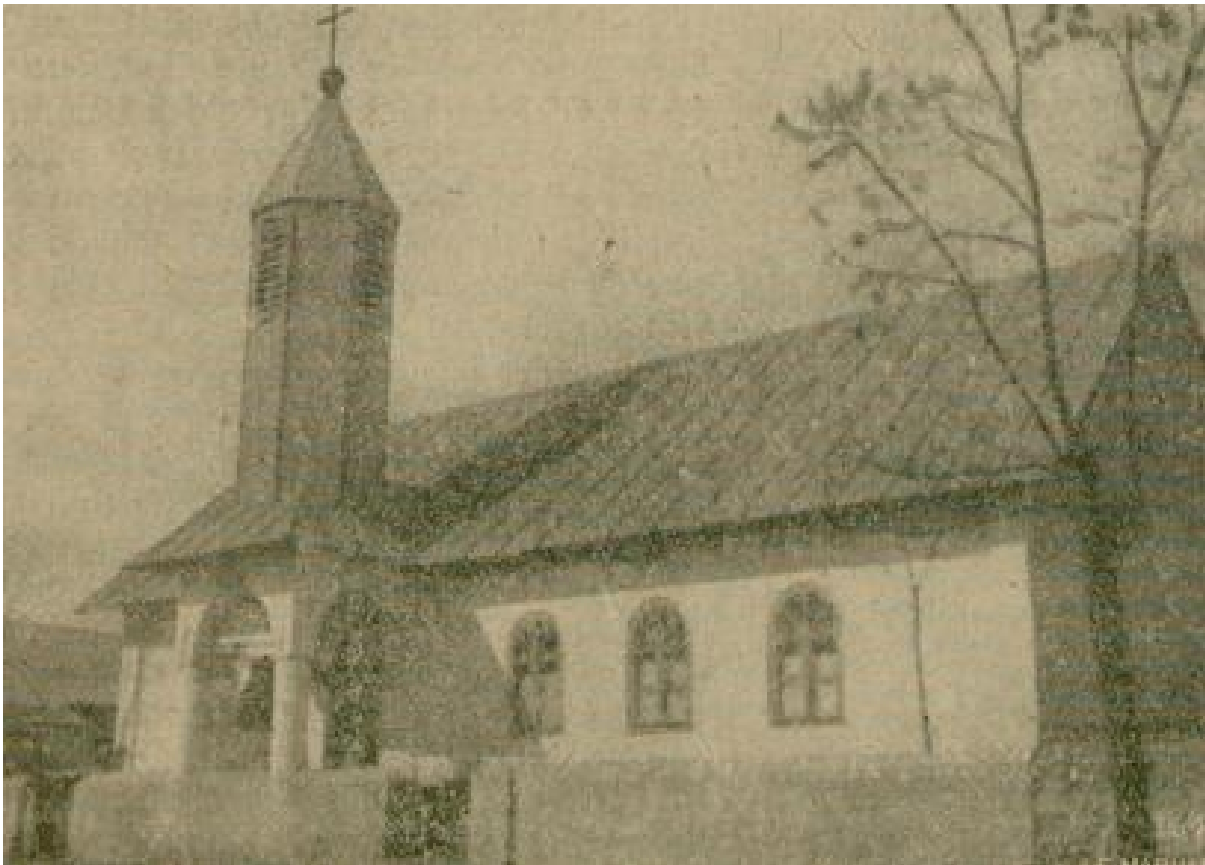
Tschukurowa Prayer House. Restored 1927
