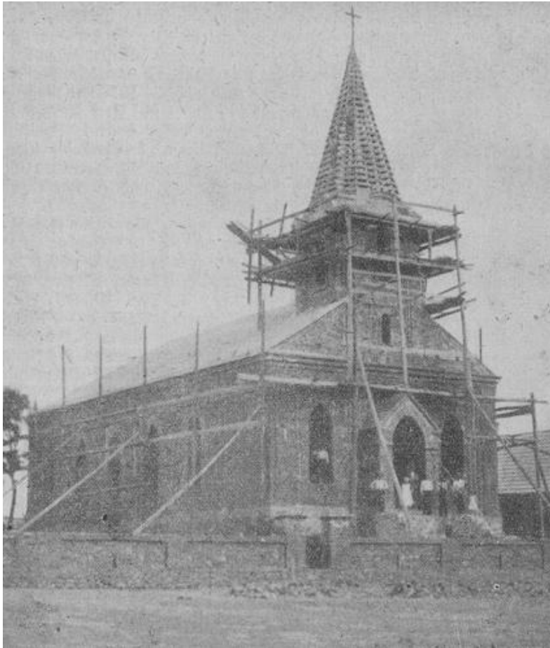
The church at Alexanderfeld (under construction)
